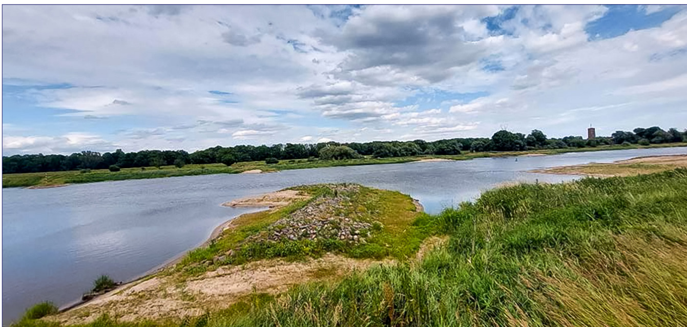
Fig. 3: Buckling-groyne with opening at low water, near Vockerode (below the A9 bridge) – Groyne opening must be lowered further, remnants of former bed reinforcement at the notch base and the landward embankment will be removed in the process.
