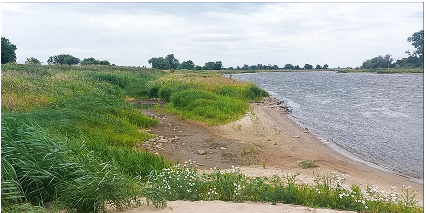
Fig. 1: Landside groyne opening near Lutherstadt Wittenberg – partially dried out at low tide but with water-filled scours, notch depth may need to be adjusted downwards.
