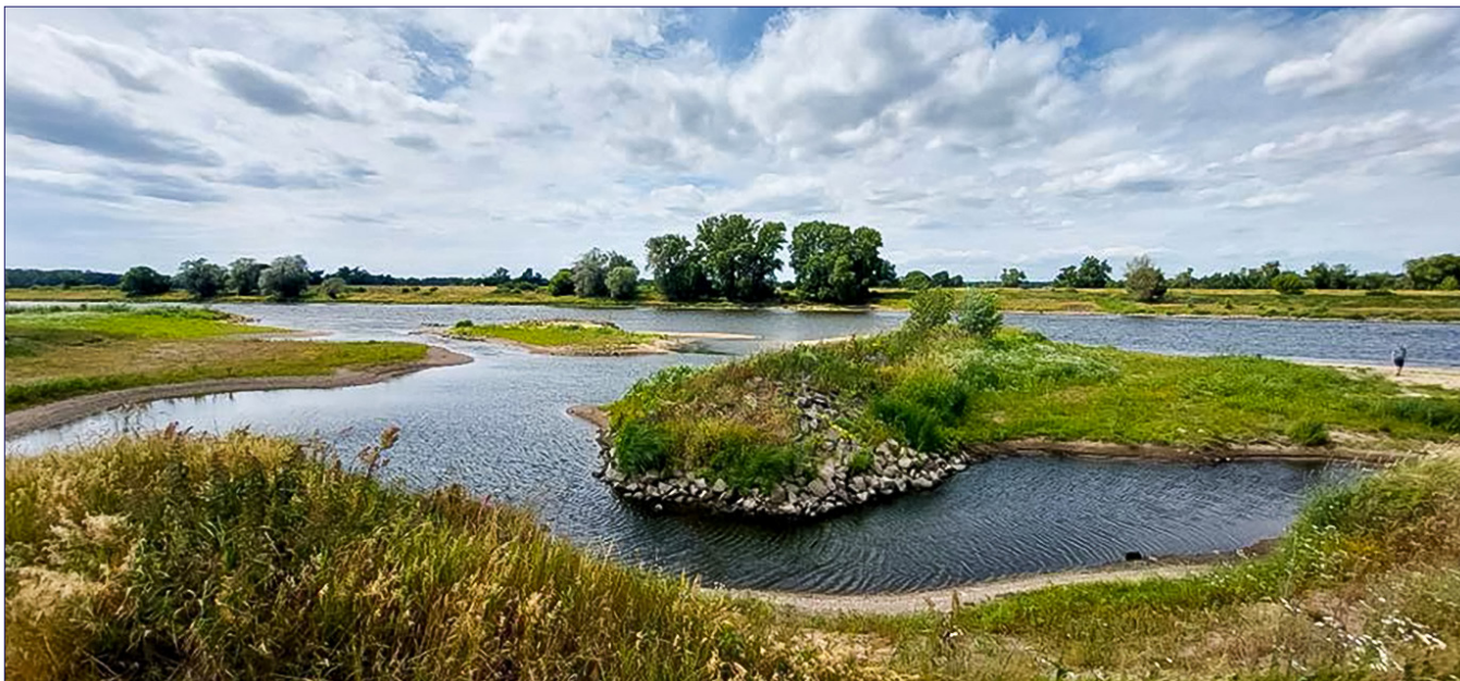
Fig. 2: Very successful groyne opening and double island-layout at low tide (near Apollensdorf/Wittenberg), regular breeding ground for oystercatchers and sandpipers.
